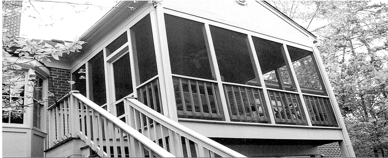
A NEW SCREEN PORCH IS ONE OF THE BEST AND LEAST EXPENSIVE WAYS TO EXPAND YOUR HOME
